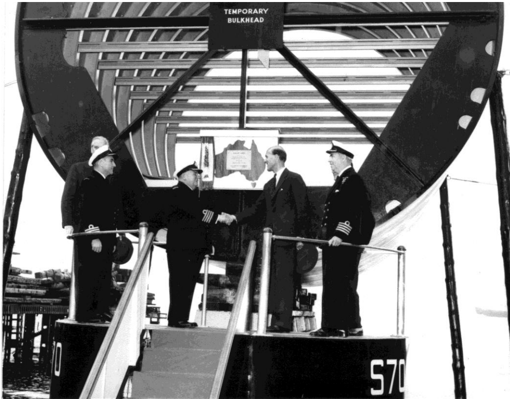
The completion of the first hull section of an Oberon-class submarine – Purves 2 nd from left presiding
